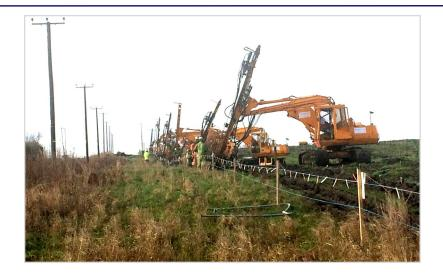
This contract was undertaken to treat extensive shallow mine workings on a greenfield site at Wellwood, North Dunfermline in advance of the infrastructure works for the first phase of a large development of up to 1100 new homes, a new primary school and a commercial development area.
